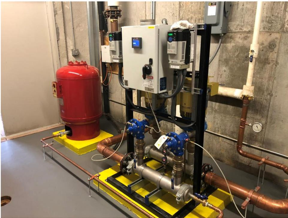
*HYFAB pressure booster with two 10-horsepower close-coupled pumps can establish the setpoint discharge for the 8-story O. Henry Hotel with as little as 14 psi of suction pressure.*
